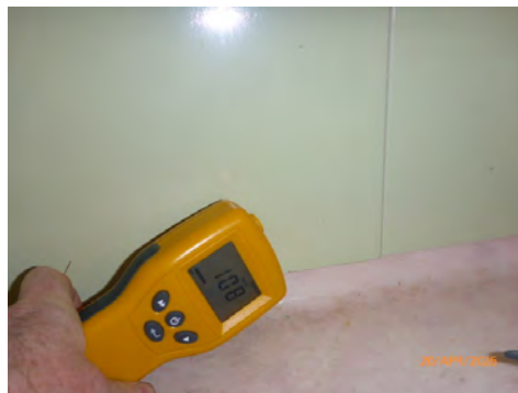
108 vegg under skyllekar
